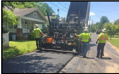
City Engineering Department repaving streets
